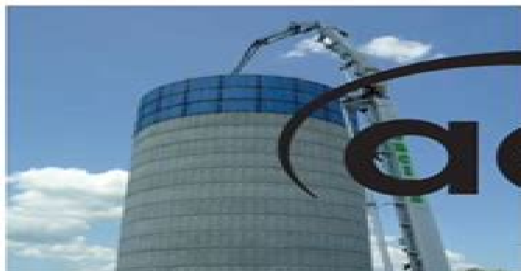
Fig. 1.4g—Construction of composite elevated tank pedestal (photo courtesy of Caldwell Tanks, Inc.).
