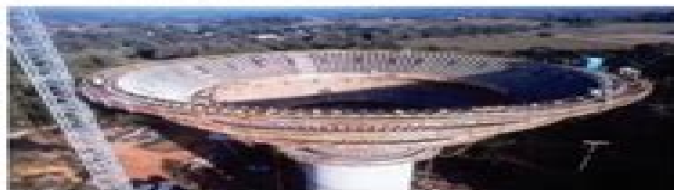
Fig. 1.4h—Construction of concrete elevated tank (photo courtesy of Cron LLC).
