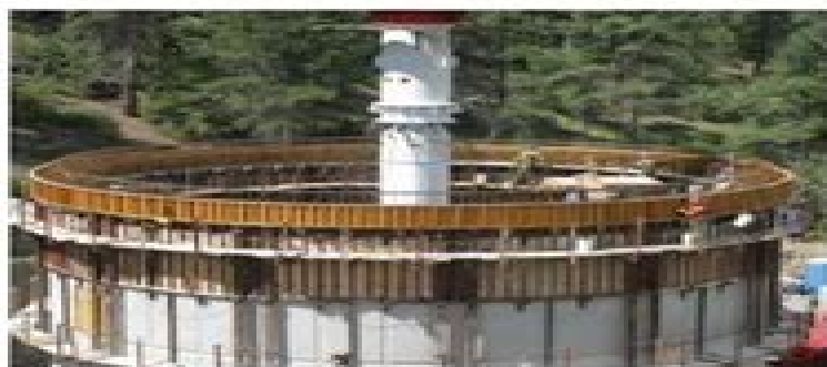
Fig. 1.4f—Construction of composite elevated tank pedestal (photo courtesy of CBI).
